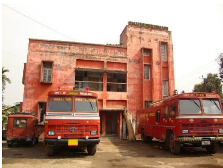
Image: Fire station at Dimapur
